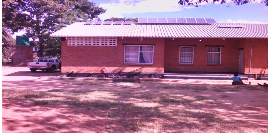
Part of the water supply system at Dzoole Health Centre
