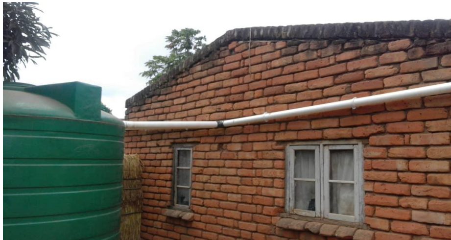
One of the rain Water Harvesting structures
