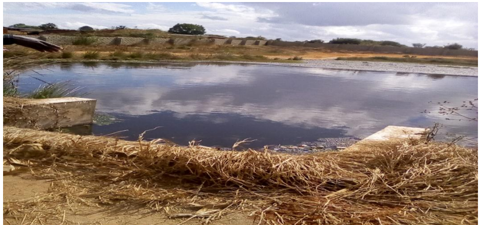
Rehabilitated Sludge Ponds at Nkhorongo, Mzuzu
